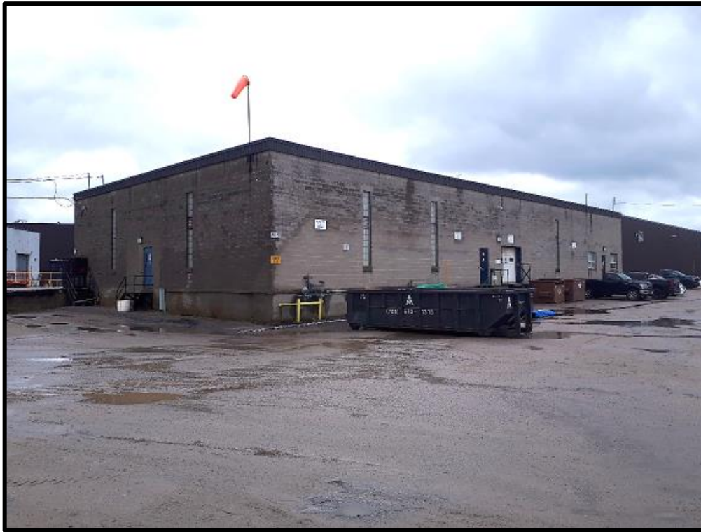
PHOTO # 1 “Old” Stores Building - North Bay
